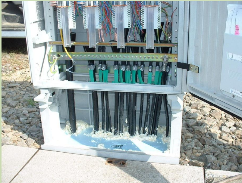
Open electrical cabinet – not yet protected against rodents –
