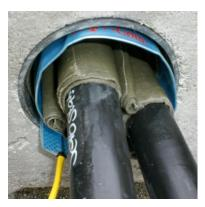
After inflation, lay valve extension in a circular position (below, left photo) or position it parallel to the cables either outside (below, middle photo) or inside (photo top right), and fix in position with insulating tape or enclose it in permanently elastic sealing tape.
